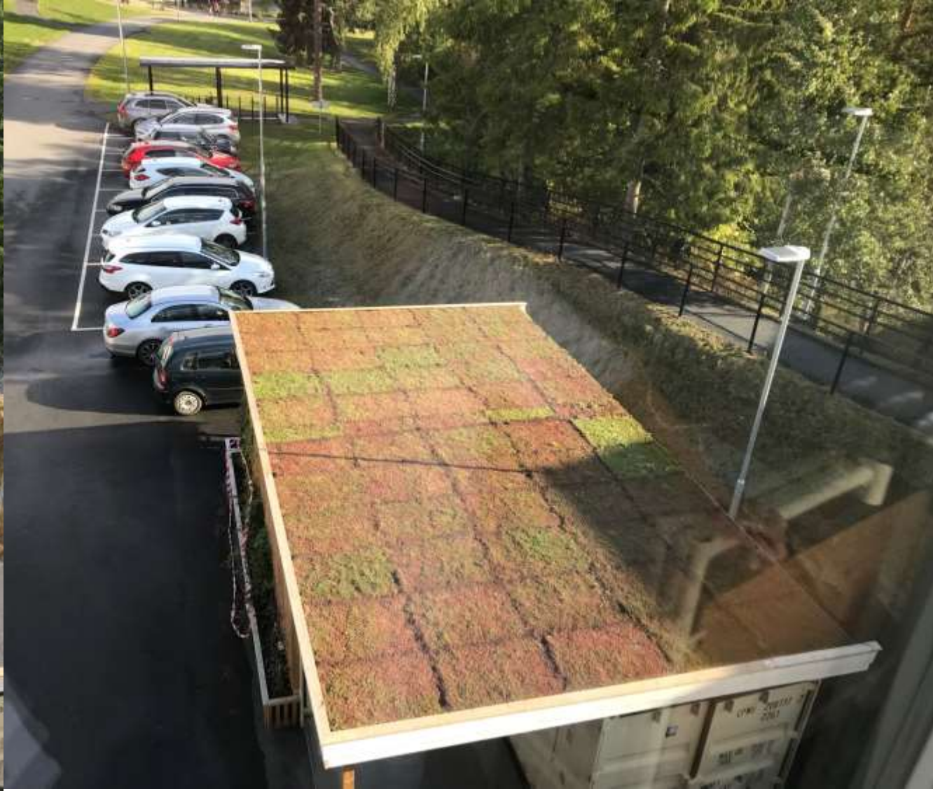
Green roof at Sunnaas newly installed fall, 2018
